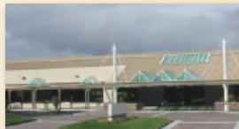
475 Oakmead Parkway, Sunnyvale, CA
